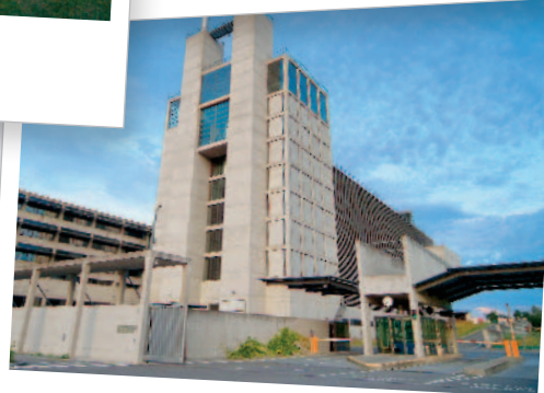
KVA Thurgau, Weinfelden
